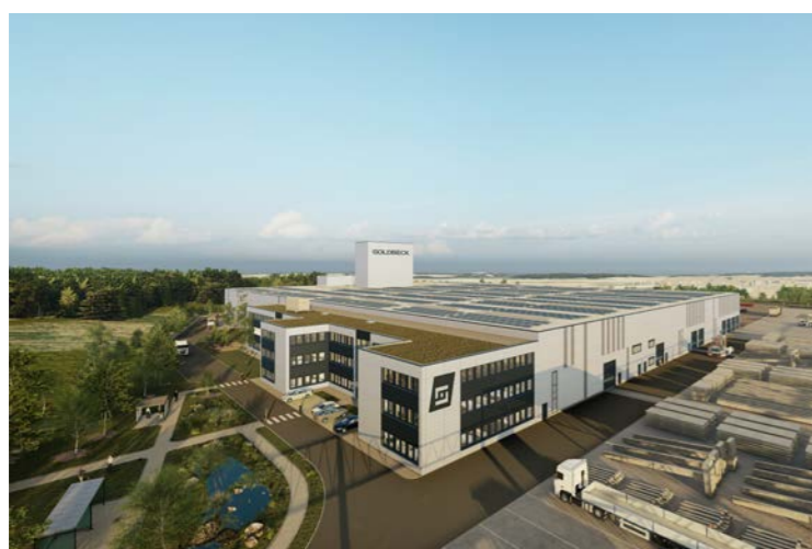
Building sustainably – for ourselves Our new plant in Kirchberg
